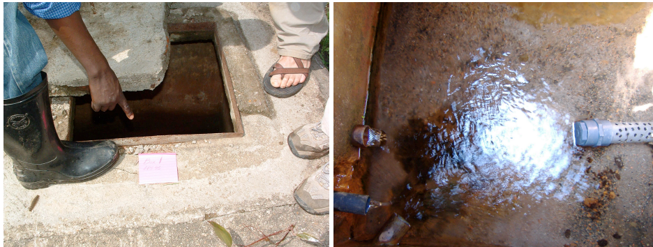
Left: External view of collection box #1. Right: Internal view of collection box #1. The pipe in the lower left corner is submerged
