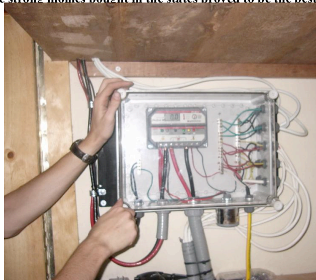
Controller mounted in closet
