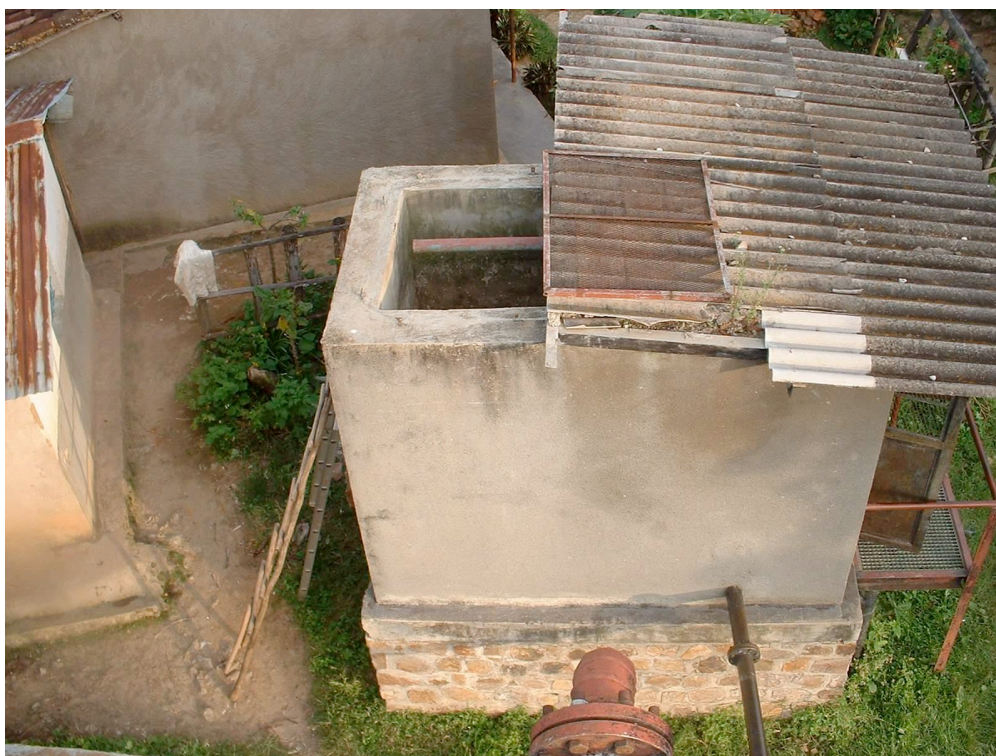
Photograph of the filter body and valve house taken from the top of the backwash tank
