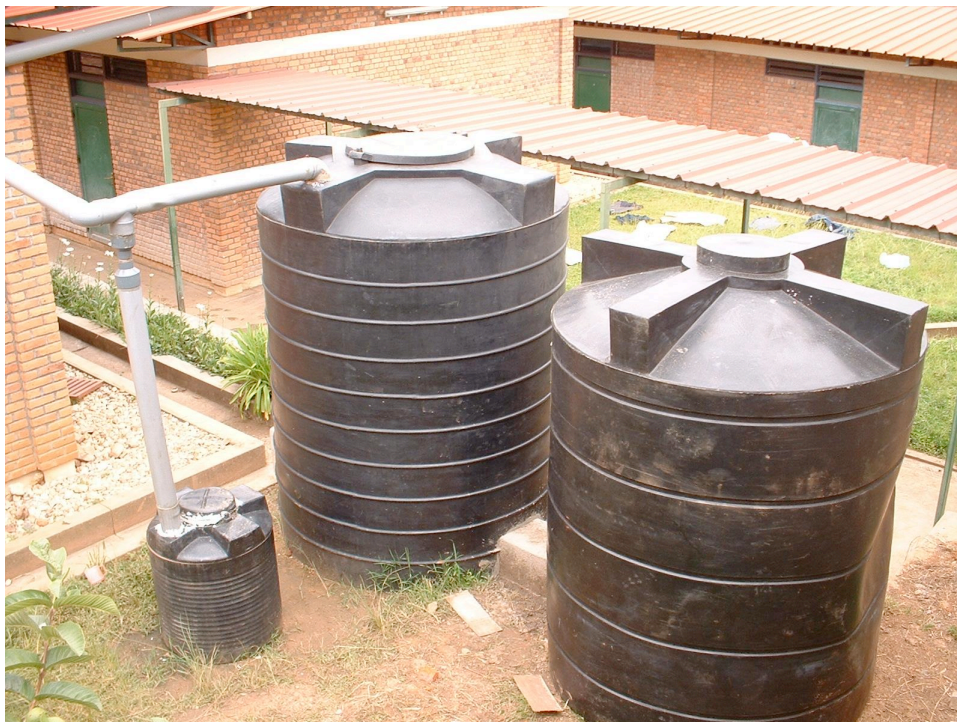
Elevated view of the expanded system. The foul flush unit is visible in the lower left corner.
