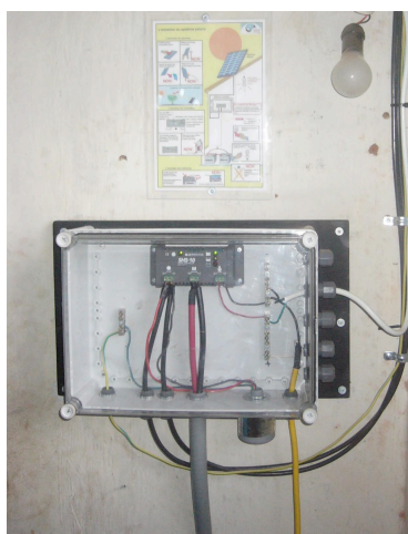
The charge controller, inside the Fibox electrical enclosure, and informational placard, located in a closet. One line ran from here to all the lights, which were wired in parallel. The battery was placed on the floor directly below this box.
