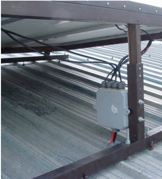
Junction box mounted to frame on roof Hole through first floor to bottom floor
