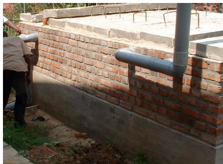
A photograph of the improper placement of the tank inlets. The inlet closest to the down-pipe is the foul flush inlet, the other one is the main tank inlet.
