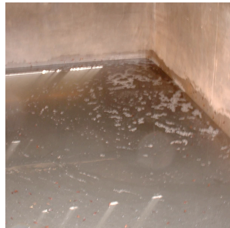
Left: A member of the team indicates the apparent high-water line in the dormitory system. The excess of dirt in the tank is a result of the foul flush being non-operational for an unknown period of time. Right: Contaminated water in the cafeteria cistern as a result of faulty foul flush construction and operation.
