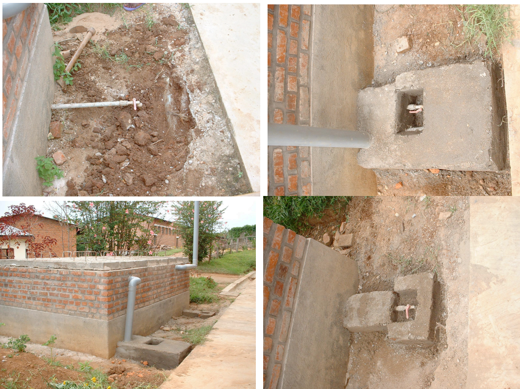
Protective masonry housings for the tank drains and the overflow pipe. The image in the upper left shows the situation prior to our improvements. The pre-existing wastewater line is buried along the edge of the concrete walkway.
