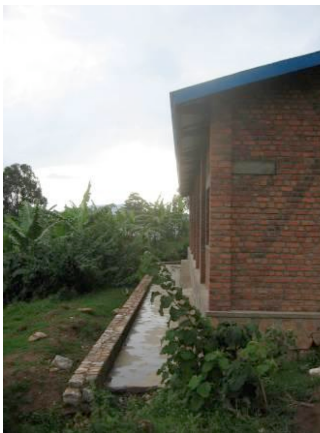
Figure 12.3.7 - The photograph below shows the ground gutter as well as the location for the collection point
