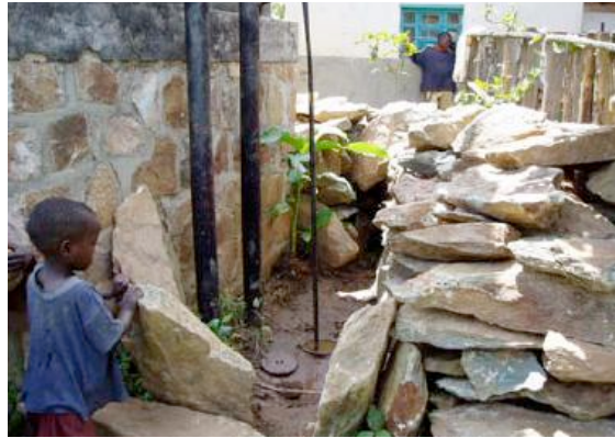
Flow diversion valve area. The valve keyhole is the hole on the ground with the metal rod sticking out. The metal rod is the valve key.
