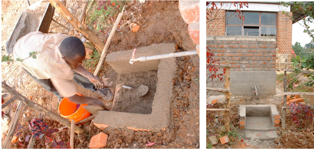
Left: JP Habanabakize applies a parge coat to the access point masonry. Right: The improved access point
