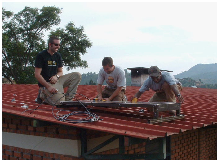
Installing the solar panel on the kitchen roof.
