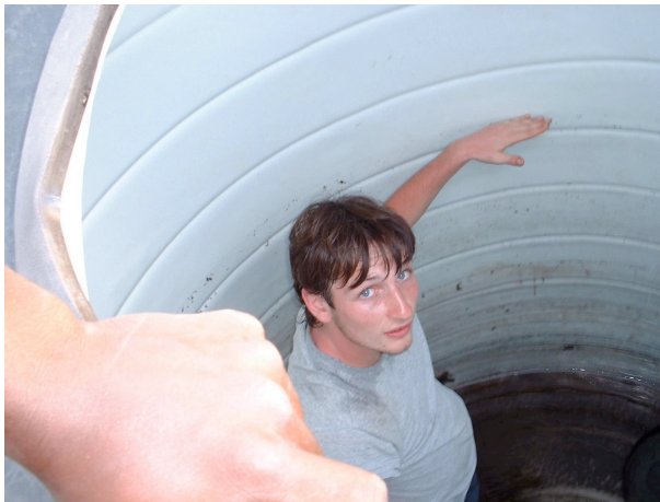
Left: A member of the team indicates the apparent high-water line in the dormitory system. The excess of dirt in the tank is a result of the foul flush being non-operational for an unknown period of time. Right: Contaminated water in the cafeteria cistern as a result of faulty foul flush construction and operation.
