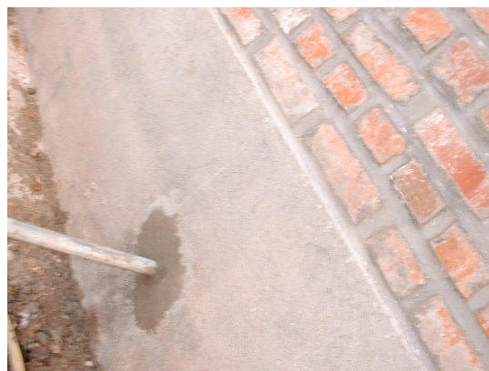
Left: Internal view of the repaired pipe-tank junction. A broom handle was used to keep cement out of the pipe while the cement hardened. Right: External view of the repaired junction
