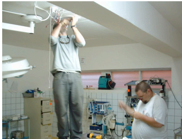
Installing a fixture in the operating room, the concrete ceilings made it very difficult to secure wires and fixtures, using the strong mollies bought in the states proved to be the best method of securing screws.
