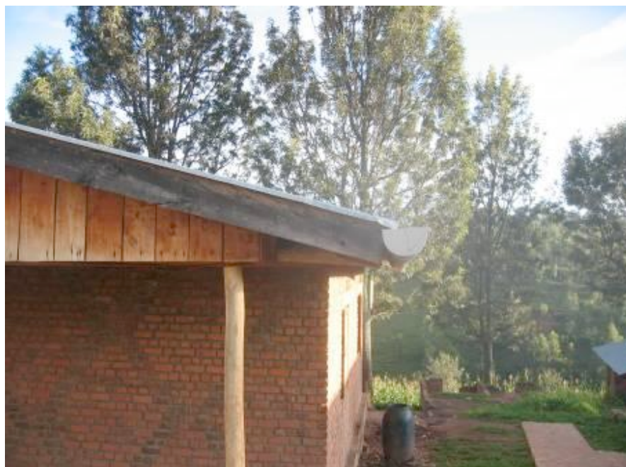
Figure 12.3.5 (Image4) – Shows the typical gutters installed on some of the homes
