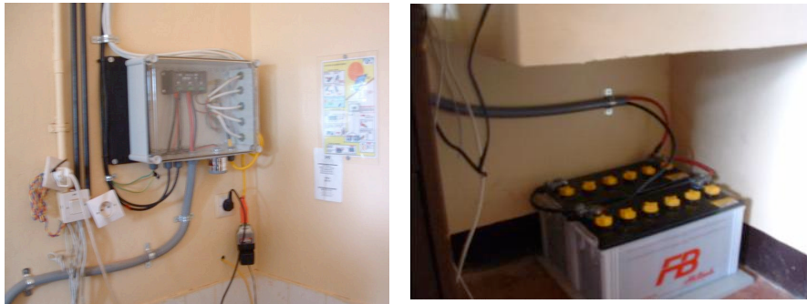
Charge controller mounted in Fibox enclosure in the computer room, yellow DC pigtail powering small inverter, Five separate lines for each light fixture.
