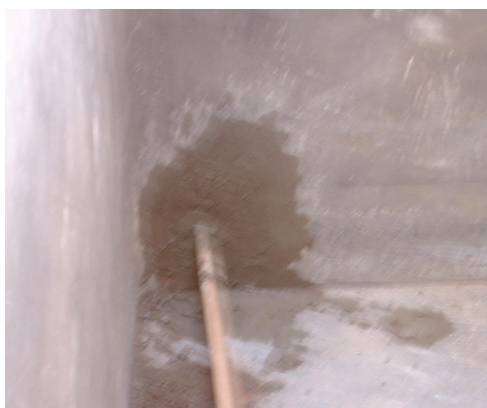
Left: Internal view of the repaired pipe-tank junction. A broom handle was used to keep cement out of the pipe while the cement hardened. Right: External view of the repaired junction
