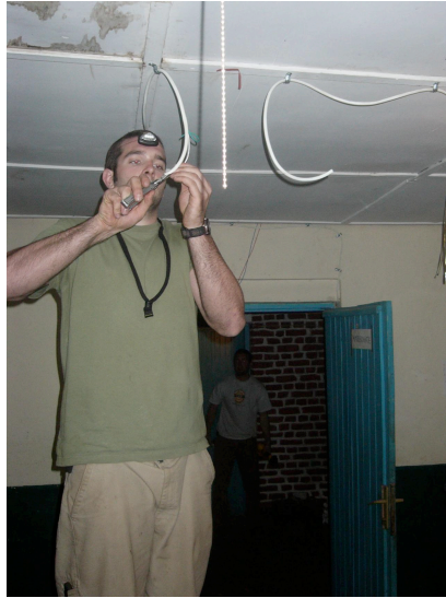
Niko installing a light fixture in the patient room. Two lights were placed in the patient room, two in the birthing room, and one under the awning at the clinic entrance.
