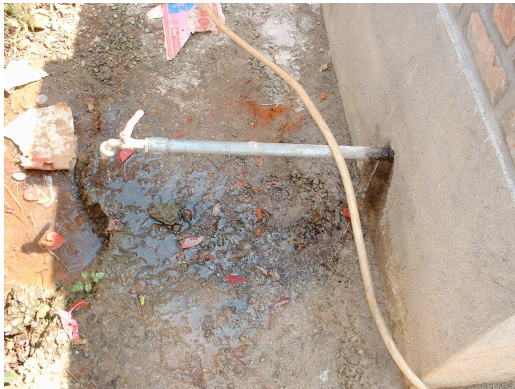
Left: Water leaking from the pipe-tank junction. Right: A photograph of the repair in progress
