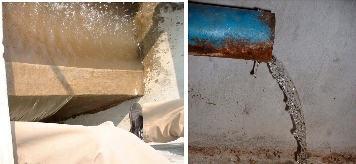
Left: Water flowing over the spillway during the initial backwash. Right: Filter effluent after the backwash. While the water looks clean, it may still be contaminated.
