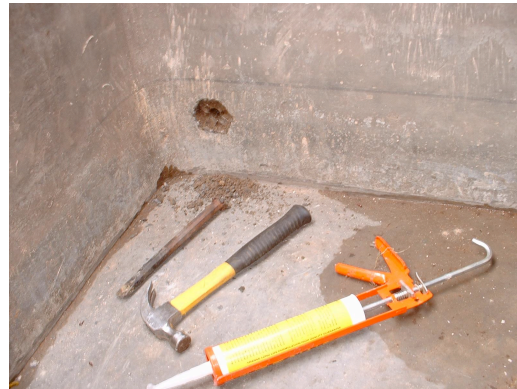
Left: Water leaking from the pipe-tank junction. Right: A photograph of the repair in progress
