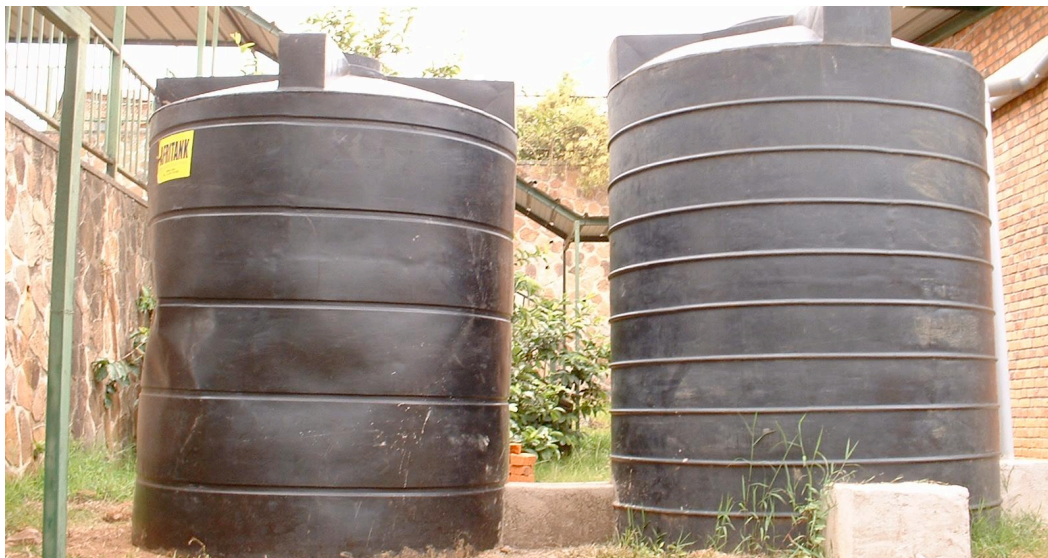
Tank junction with masonry housing. The new tank is on the left and the old tank is on the right. The dents in the new tank were caused during transport and will disappear when the tank is filled for the first time. The masonry boxes in the lower right corner are the tap and drain housings.
